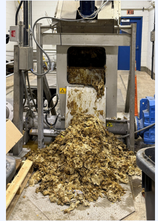
Clog at Stayton Wastewater Treatment Plant due to wipes
