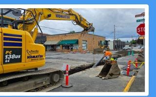
and the addition of new valves to reduce the impacts of future water shutdowns. Two (2) ADA compliant curb ramps have been constructed, and demolition has begun for the lowering of the curb and sidewalk on the south side of Ida St. between 2nd and 3rd Ave.
