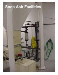
input signal from the filtered water flowmeter. Water to make a soda ash solution is added to the tank through a simple float valve, which maintains the tank at a predetermined level.
