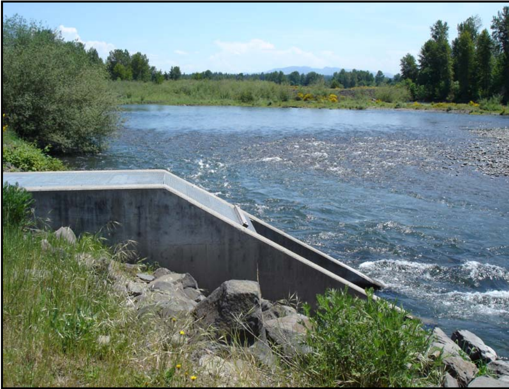
Photo 13: Viewing Platform Site at Fish Screen Bypass
