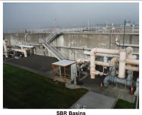
Basin mixing is performed by two headers in each basin and an external 125 HP centrifugal pump, one for each basin. Aeration is accomplished using two (2) 200 HP K-Turbo blowers (now owned by Aerzen)
