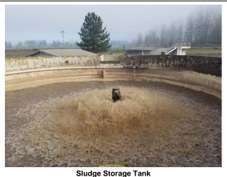
Storage Tank #1. The sludge storage pond is concrete lined and according to City staff needs repair.
