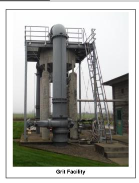
Pumped grit is sent to the grit cyclone/classifier which dewaters the grit and deposits it into a dumpster. The grit removal system is operated by a timer system. A flush valve is opened periodically to fluidize the accumulated grit in the bottom of the vortex grit chamber to allow easier removal. The City staff report the solenoid flush valve had been having issues and was replaced in November 2019.
