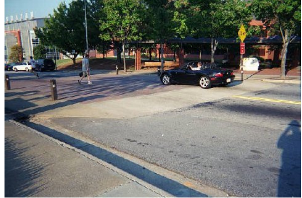
Raised intersections and changes in materials at gateways can improve pedestrian crossing safety and reduce traffic speeds.
