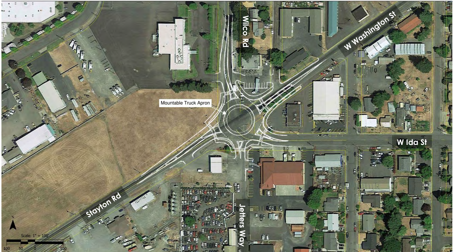
Figure 12. Stayton Road SE / Wilco Road Roundabout
